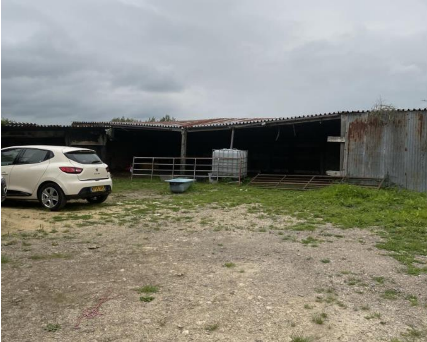
Corrugated metal building running along northern boundary
